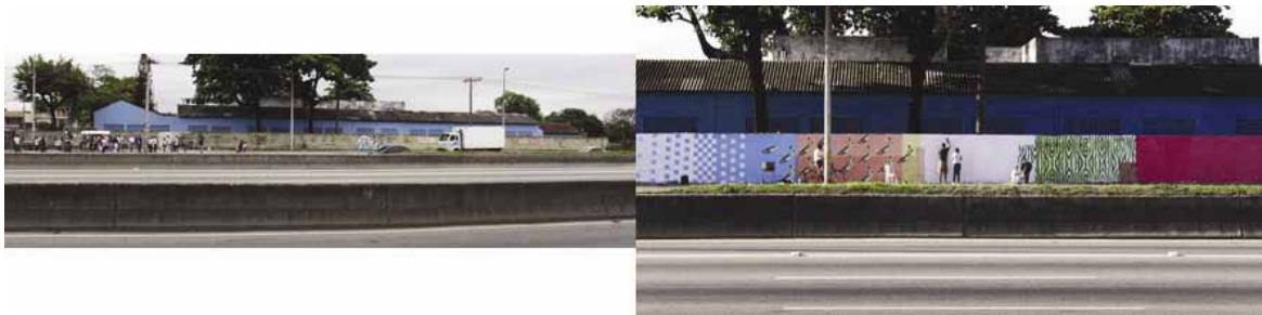
Figure 1. View of the wall from Avenida Brasil, before and during the intervention.
